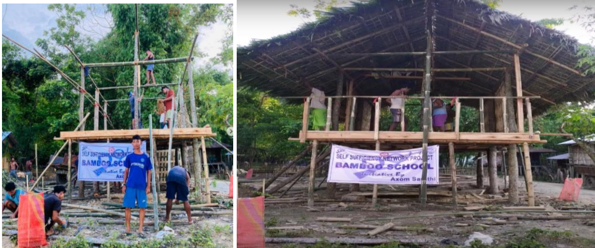
Figure 5 Construction of the Bamboo School House by the Village Youth
